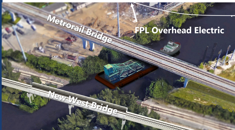
Float Out Bascule Demolition
