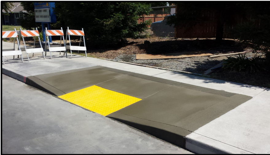
Example of Curb Ramp Reconstruction
