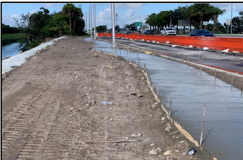
Sidewalk is poured for eastbound Southern Boulevard. October 2020
