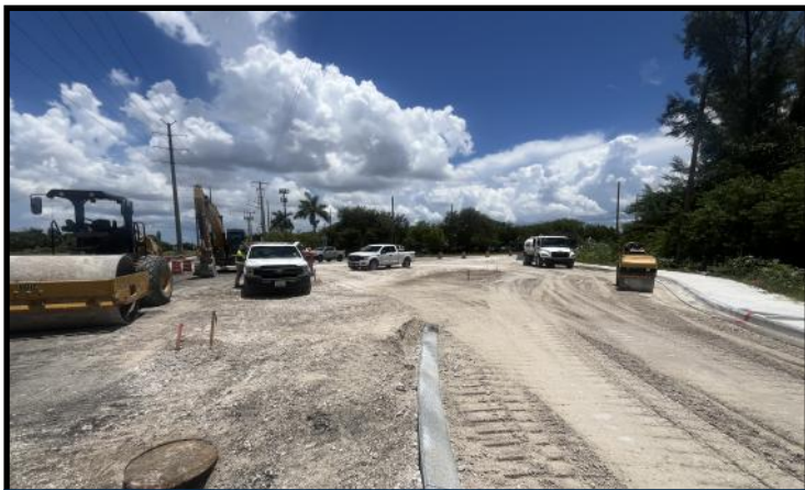
Parkside Drive Roundabout Construction
