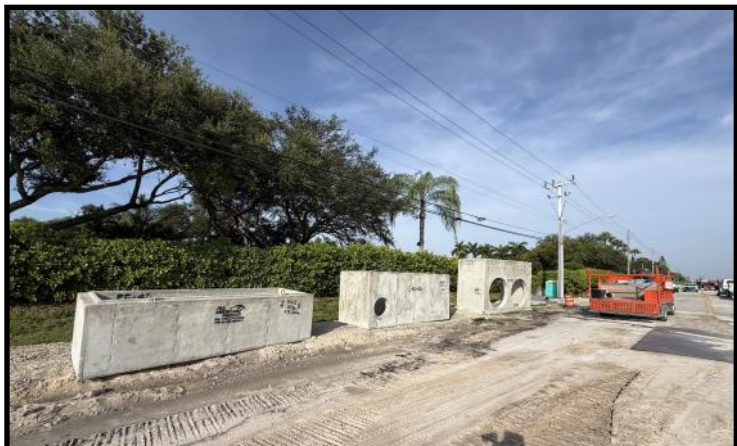
Drainage Structures East of NW 61 st Way
