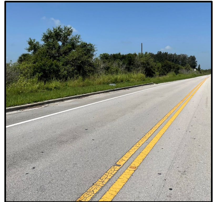
Westbound CR 606/Oslo Road (pre-construction)
