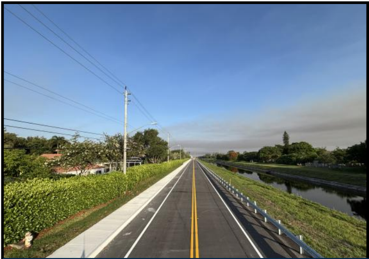
Completed Phased Work West of NW 61 st Way
