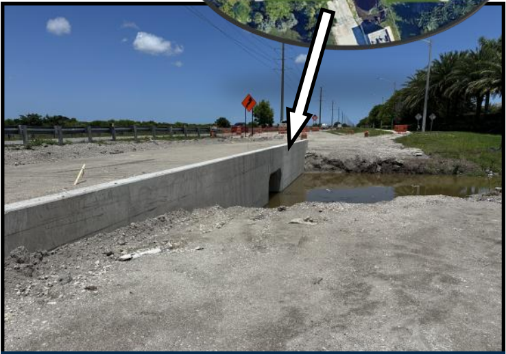
Box Culvert Installation
