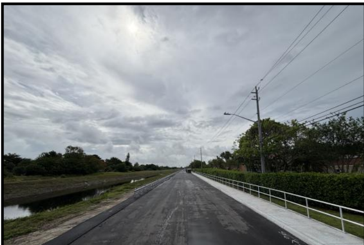
Sidewalk Installation from Parkside Drive to NW 61 st Way
