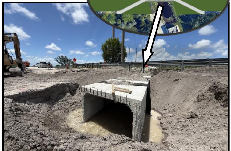
Box Culvert Installation
