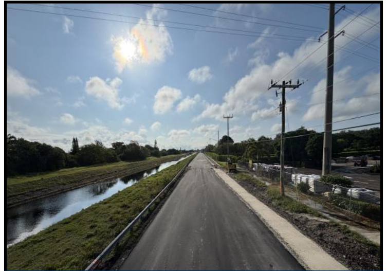
Asphalt Installation East of Parkside Drive
