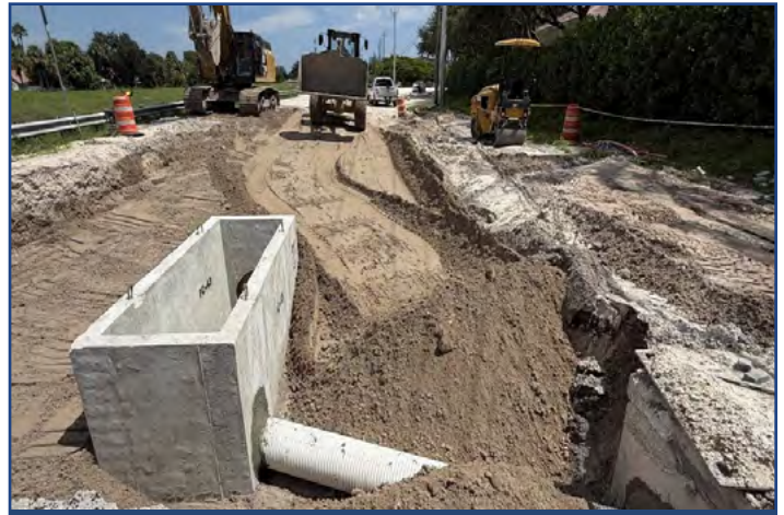
Drainage Installation east of NW 61 st Way
