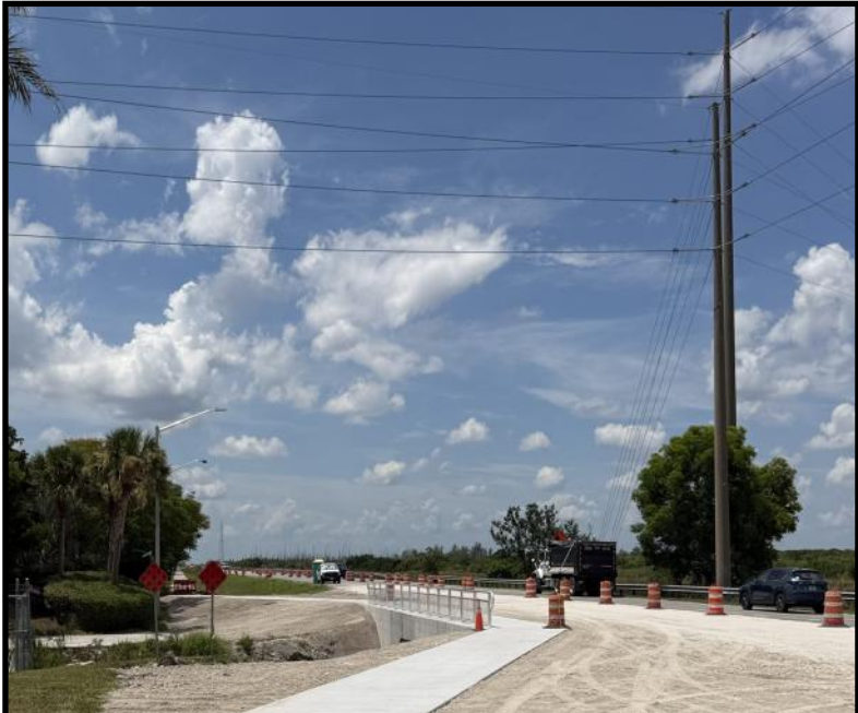
Box Culvert Sidewalk Installation
