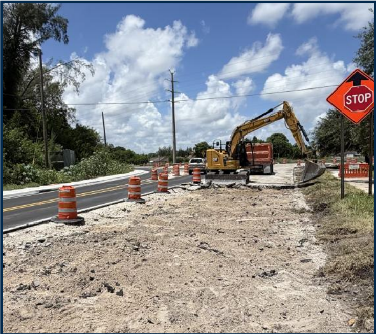
Parkside Drive Roundabout Construction
