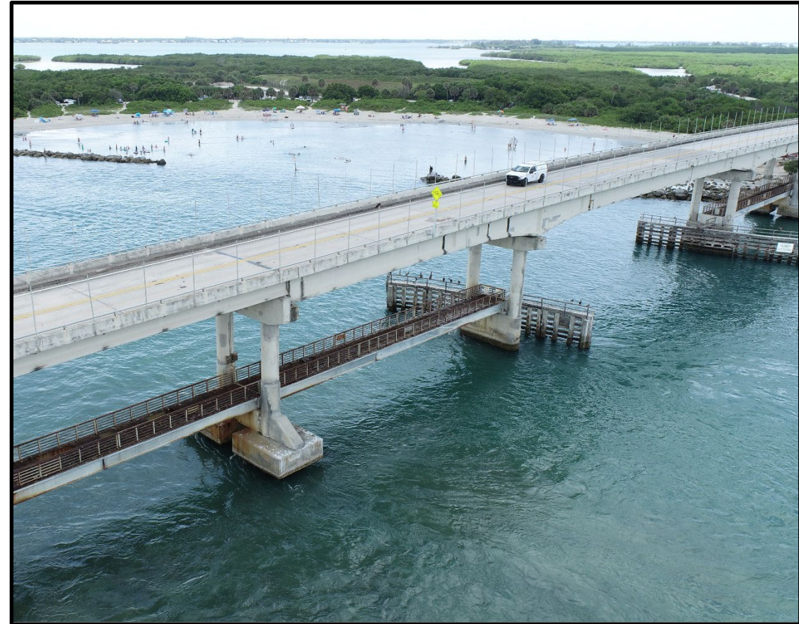
Existing S.R. A1A/Jimmy Buffett Memorial Highway over Sebastian Inlet Bridge and Observation Decks (Pre-Construction)
