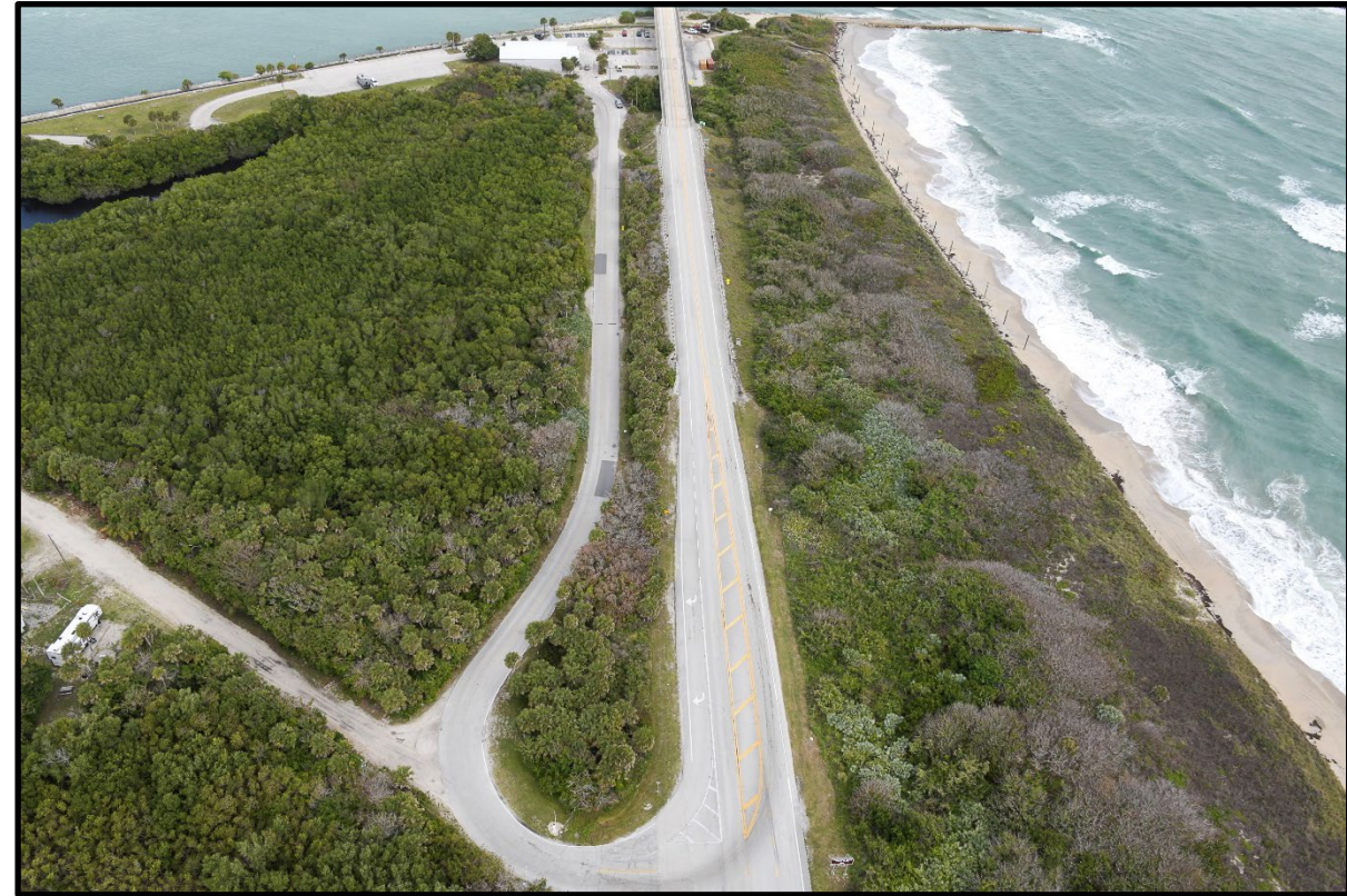
Existing S.R. A1A/Jimmy Buffett Memorial Highway and the south entrance to the Sebastian Inlet State Park (Pre-Construction)
